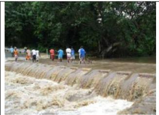
Epau Villagers walk across the recently reconstructed Epau River Crossing during the recent flood. After the waters receded, the structure was found to be undamaged.
